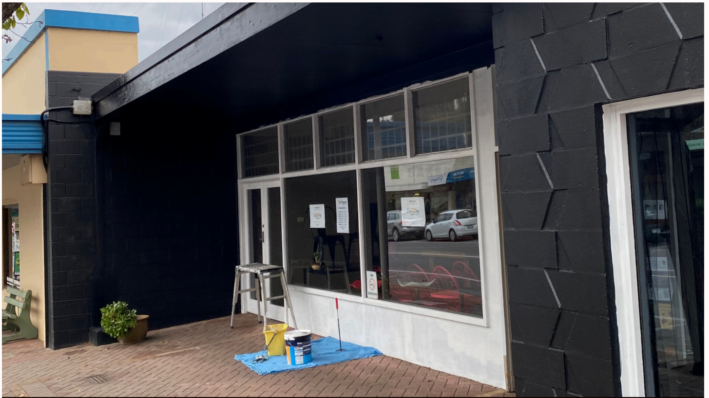
MANNUM STORE RENOS UNDERWAY
