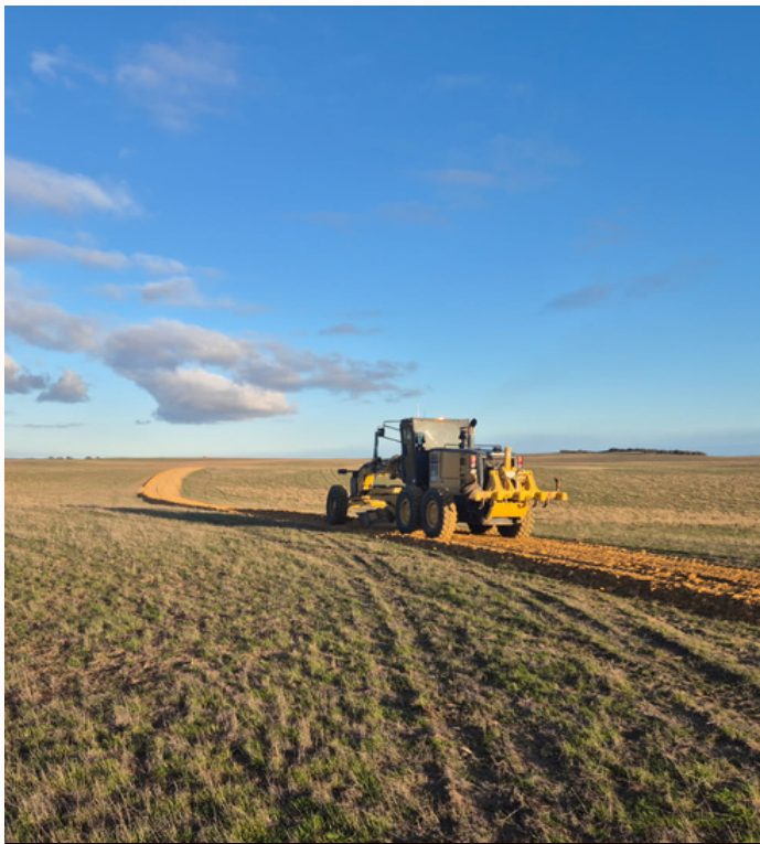
GRADER IN ACTION BUILDING FARM TRACKS
