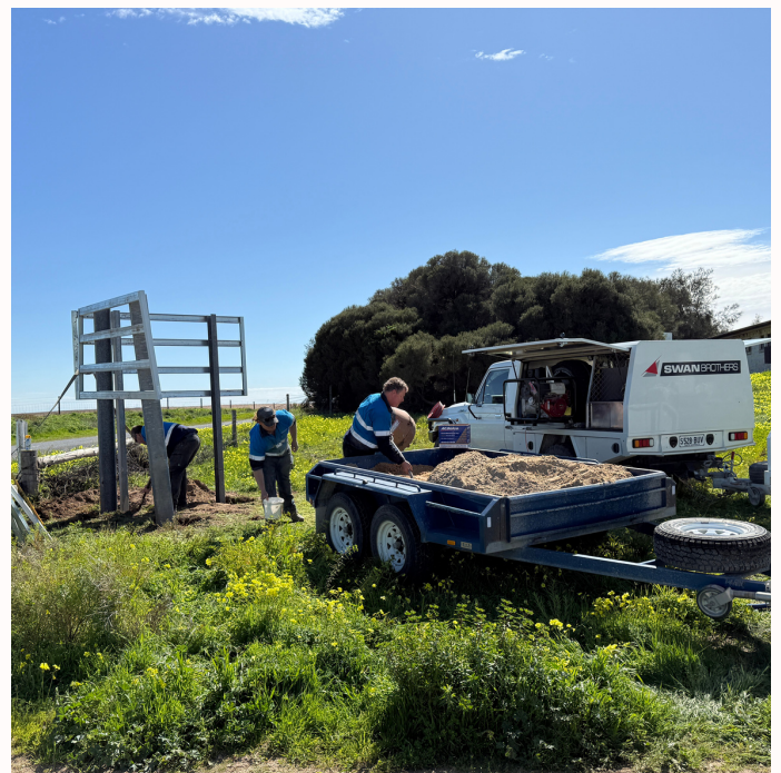
SHM INSTALLING THE FRAMES
