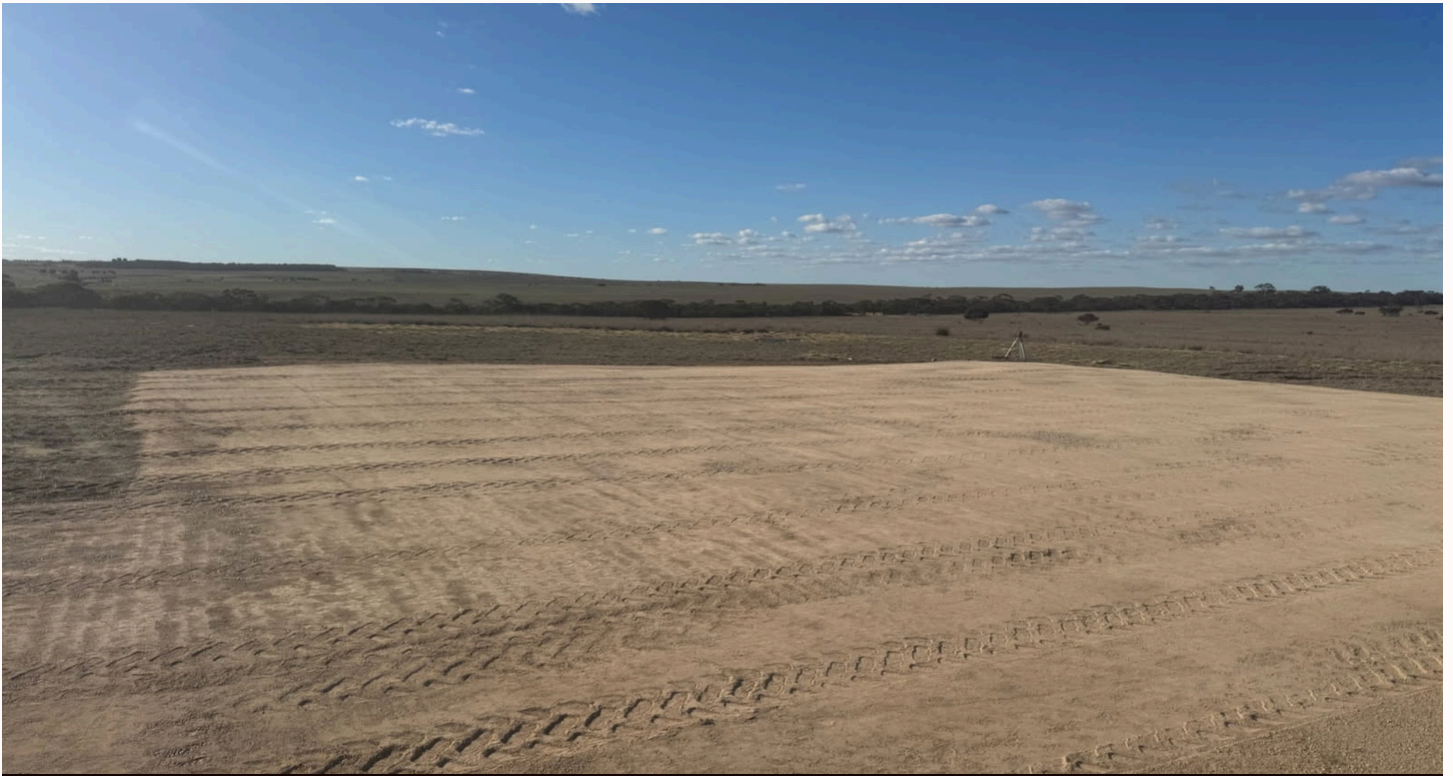
A COMPLETED SHED PAD
