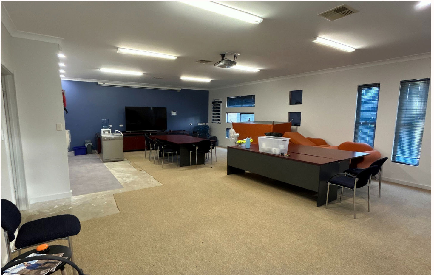
BOARDROOM RENO PROGRESS PHOTO
