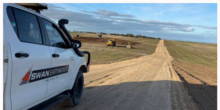
NEW TRACKS IN USE
