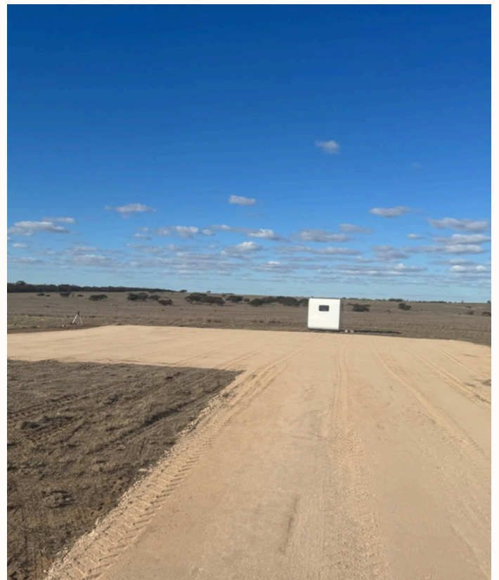
SHED PAD AND TRACK
