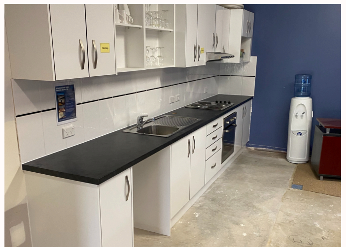
KITCHEN RENO PROGRESS
